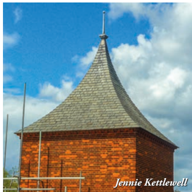
Delabole tiles on the lower roof
